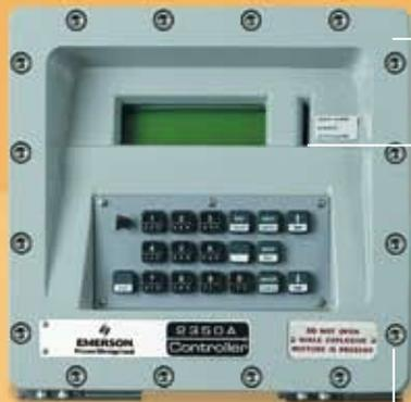
Optional explosion-proof housing allows for operation and diagnostics to be performed in a Class I, Division 1 hazardous area.
