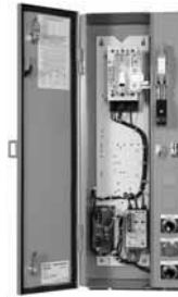
Type 12 Combination IT Starter with HMCP
