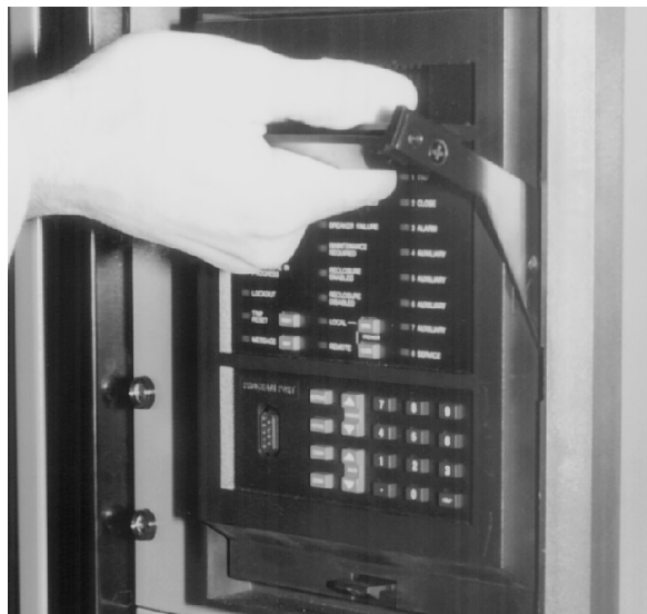
Figure 3-6: ROTATING HANDLE TO STOP POSITION
