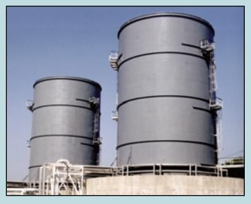
The ZTOF flare design has been used to provide up to 200 ton/hr enclosed flare capacity in a dual unit enclosure design.
