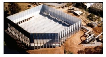
The LRGO multi-burner flare system can be provided with radiation fences that completely shield the flame visibility and radiation at grade.
