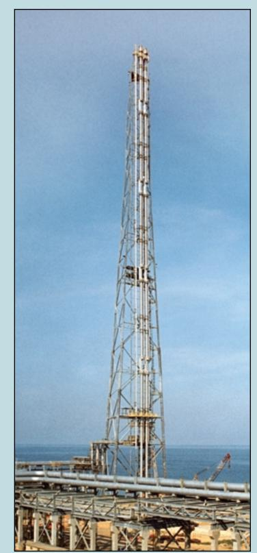
John Zink's demountable derrick structures allow multiple flares to be installed on a common structure. The demountable design allows the individual flare tips to be lowered to grade while the other flares remain safely in service.
