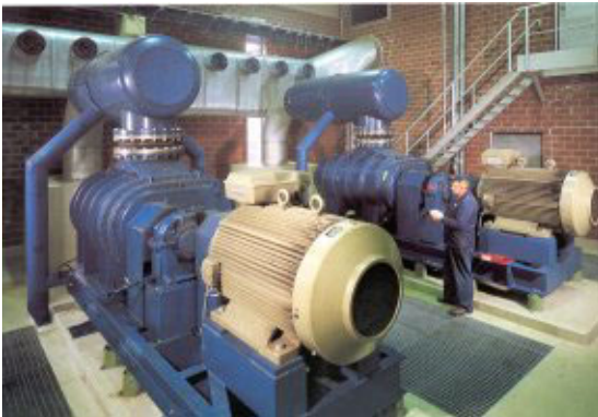
Application with a compressor
